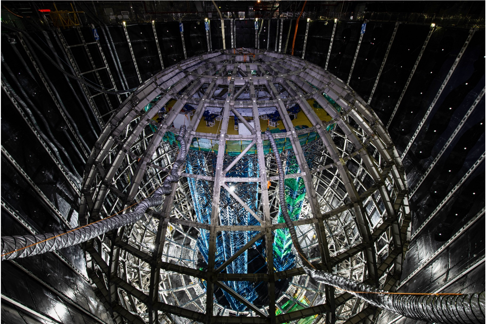
Real photo of the stainless steel structure inside the water pool. Picture taken on November 2022.
